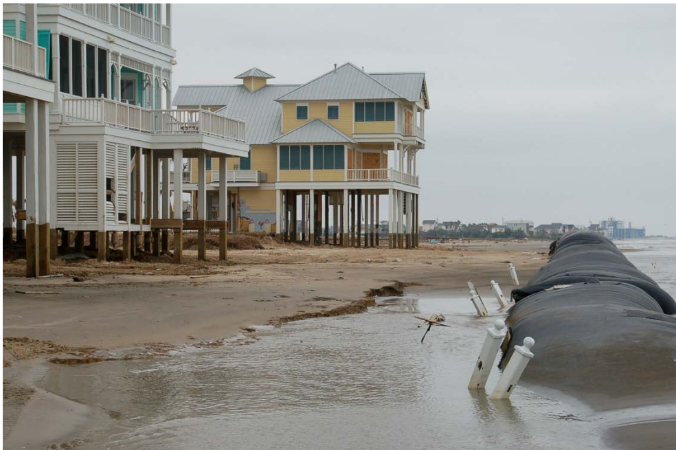
Figure 4. Erosion along the Galveston Island shoreline, west of the seawall (Oct. 17, 2008, photo C.P. Jones)
